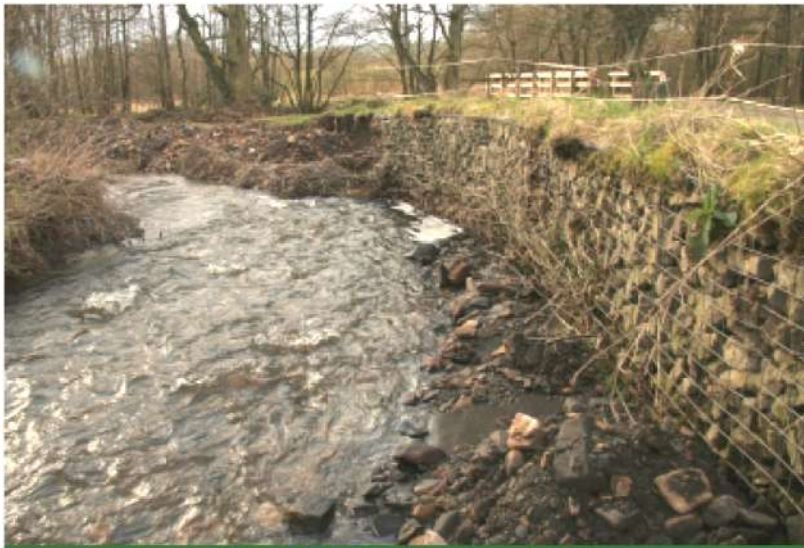
View of the collapsing gabions in 2008
