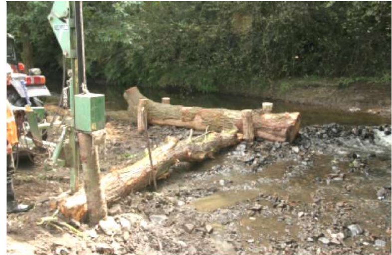
The 'Key Piece' of the ELJ was a 5 tonne oak tree trunk. This was 'keyed' into river bed and supported with oak posts driven deep into the substrate. Further strength was created by adding a 'T piece'.
