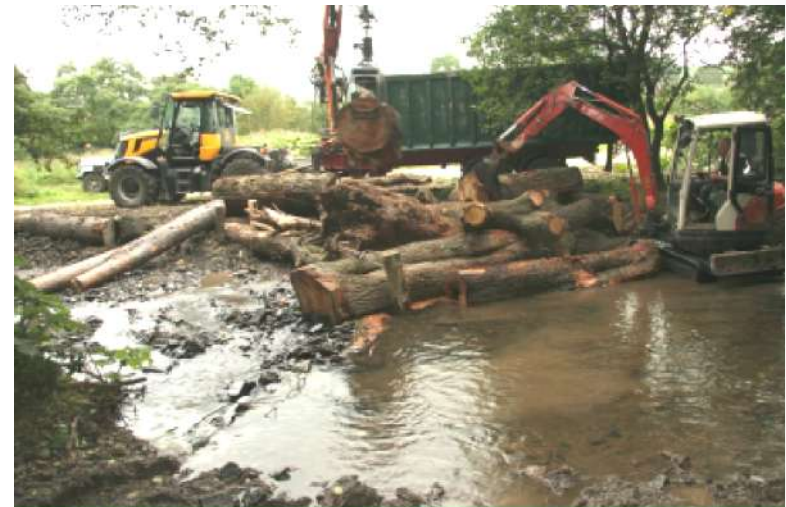
A further 22 tonnes of trunks and root plates were used to construct the ELJ.
