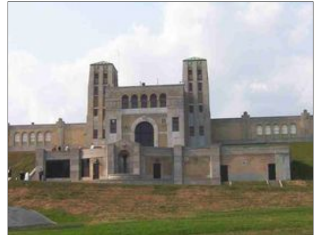
R. C. Harris Water Treatment Plant, Toronto
